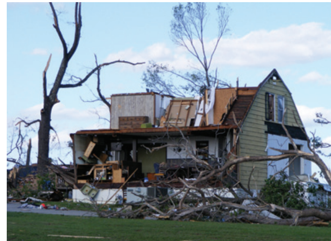
▼ Damaged house in Pleasant Grove
